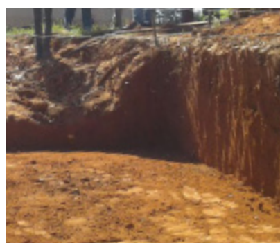
Canal: 1 Length: 10.5 m Width: 5 m Depth: 0.9 m
