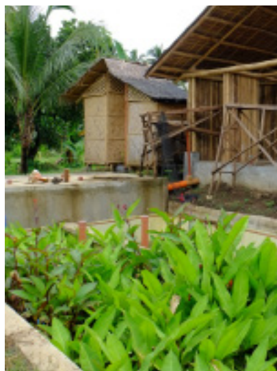
Horizontal subsurface flow constructed wetland.
