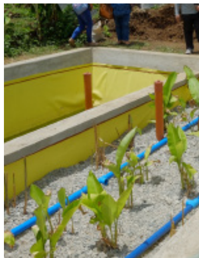
Vertical subsurface flow constructed wetlands.
