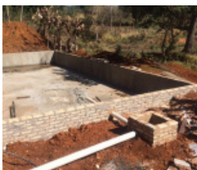
Canal: 1 Length: 12 m Width: 4.5 m Depth: 0.9 m
